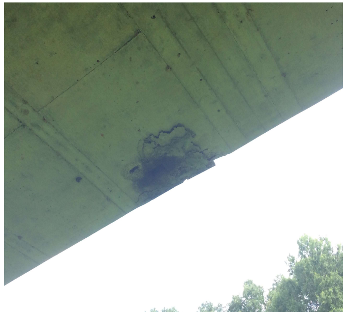
PHOTO 2 Description Spall and delam span 5 right side
