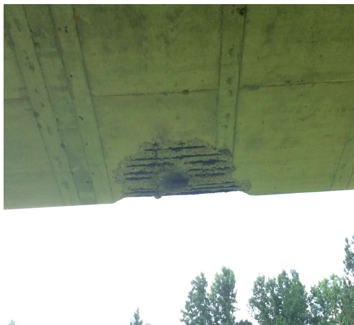
PHOTO 3 Description Spall with rebar exposed left side span 4
