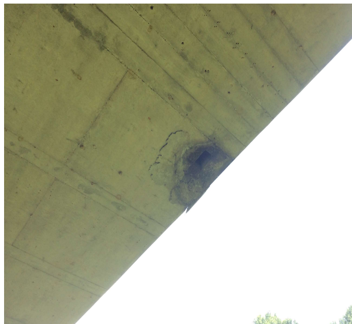
PHOTO 6 Description Span 2 right side delam bottom of slab
