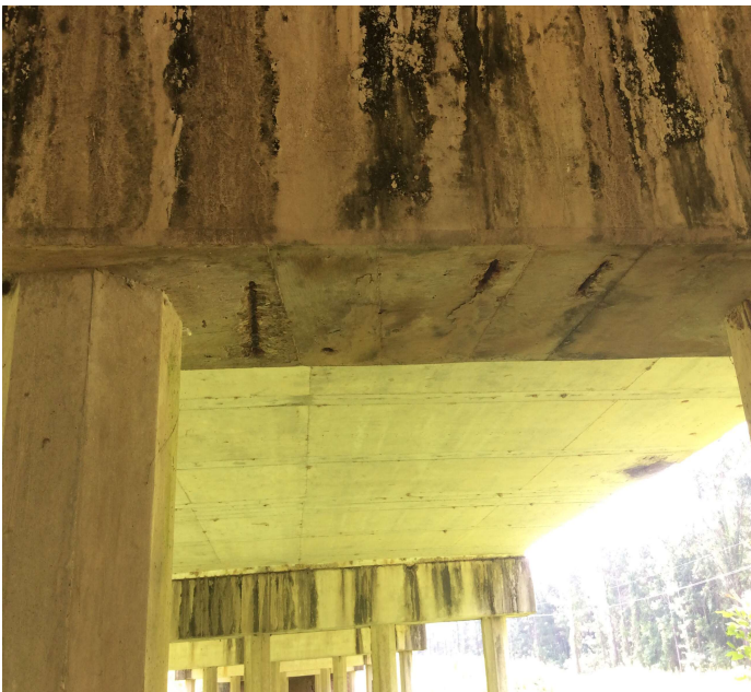
PHOTO 1 Description Spalls bottom of bent 6 cap
