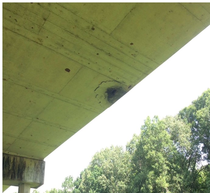
PHOTO 5 Description Span 3 right side delam bottom of slab
