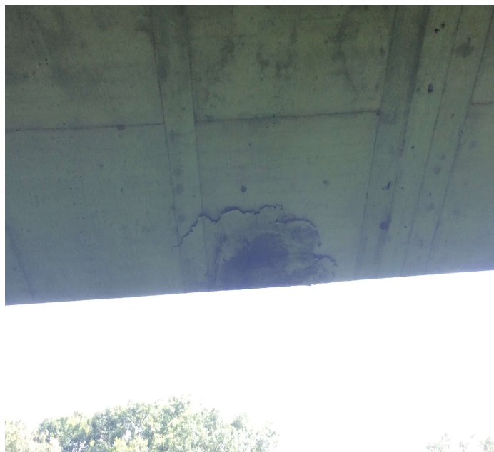
PHOTO 4 Description Delam right side span 4
