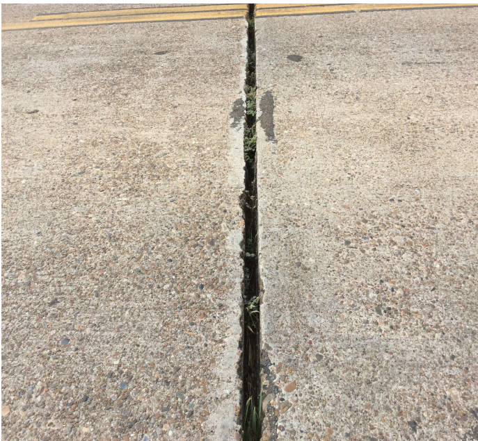
PHOTO 1 Description All joints need cleaned and refilled
