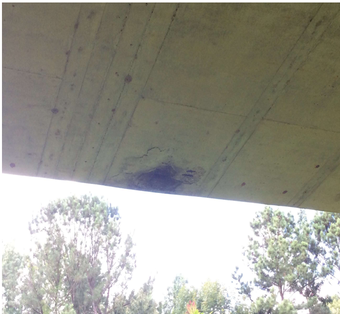
PHOTO 1 Description Span 5 delam and spall bottom of slab left side
